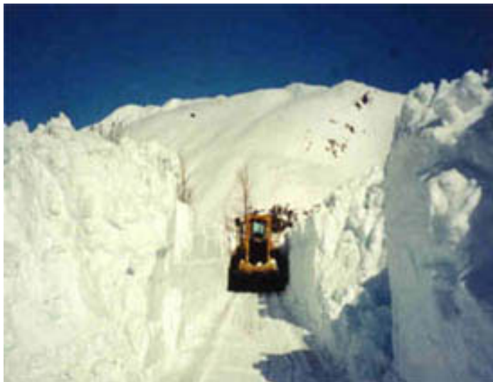
Figure 5: A picture after heavy snowfall during the tunnel reconstruction
