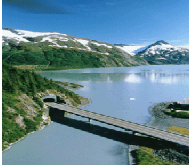
Figure 1: A view of the new bridge and tunnel
