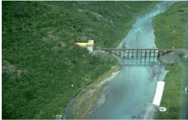
Figure 3: One side of the tunnel and a new bridge
