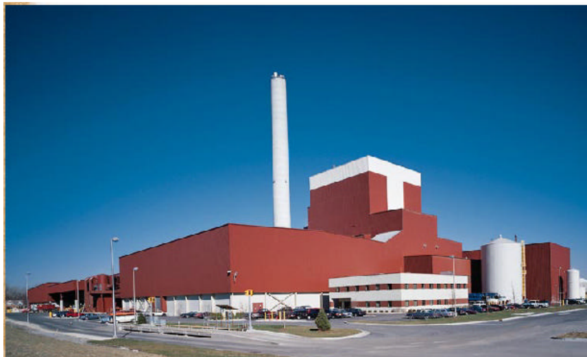
Figure 9. The Robbins waste-to-energy facility near Chicago. This plant utilizes presorting, modern circulating fluidized bed furnaces and comprehensive air pollution control technology to achieve extremely high environmental performance (Foster-Wheeler (1998)).
