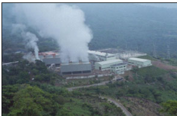
Figure 3 - Berlín Power Plant
