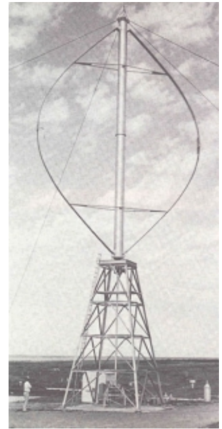
Figure 2-4: Darrieus rotor used for irrigation in Bushland, TX. From Park 1981
