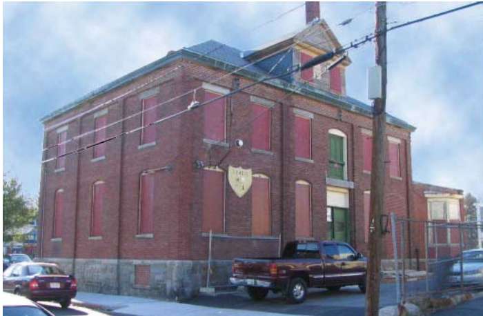
Figure 17: the northern facade of the former Parks and Recreation building on Hampshire Street Current Conditions:
