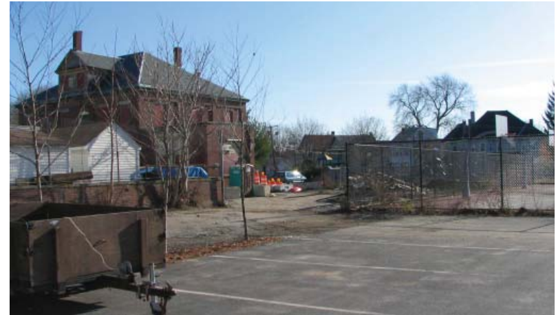
Figure 18: from the parking lot on Jewett Street, orange barrels and piles of fill are visible in the parking lot.
