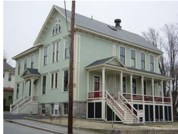
Figure 23: the Tenth Street School after renovation, now contains two residential condos
