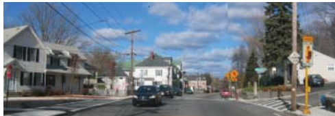
Figure 14: The intersection of Hampshire Street and Jewett Street at Bridge Street
