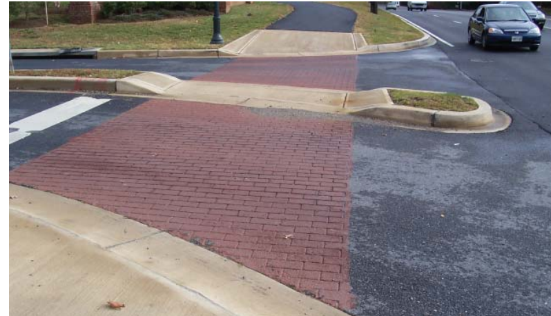
Figure 1: Crosswalk stamped to resemble brick.
