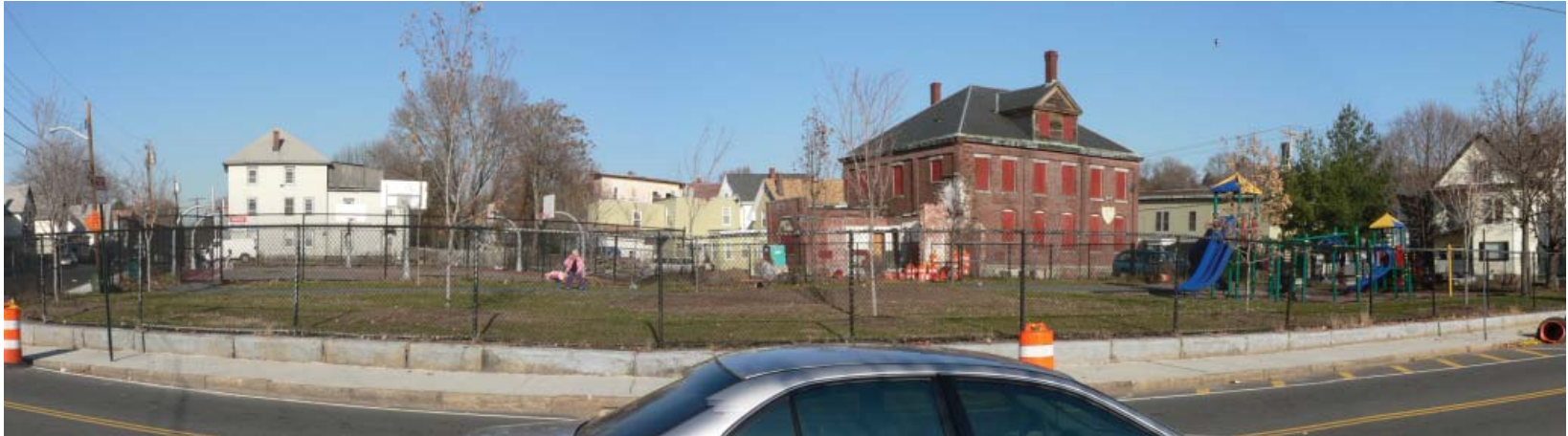
Figure 13: currently, the playground is completely fenced off from West Sixth Street
