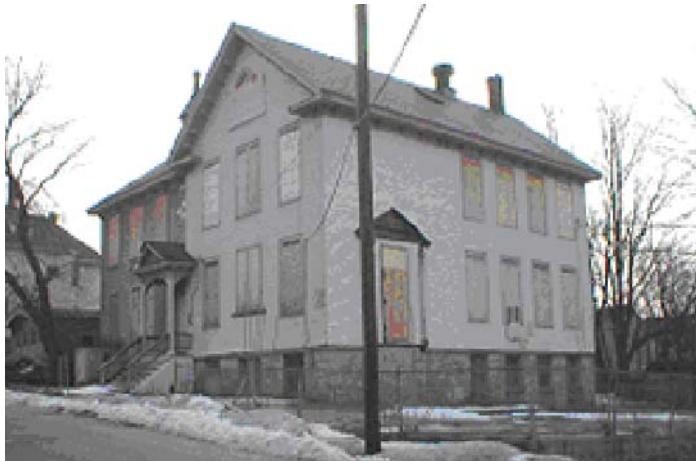
Figure 22: the Tenth Street School before renovation
