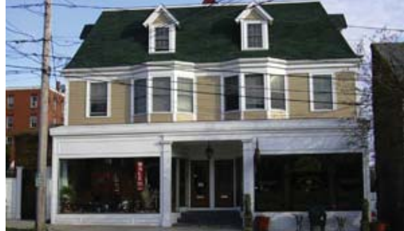
Figure 12: typology of building possibly suitable for infill at 84 West Sixth Street
