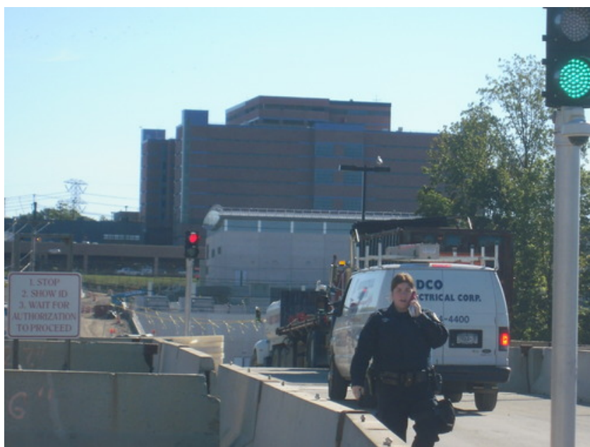
Above, the plant during final construction and testing last year.
