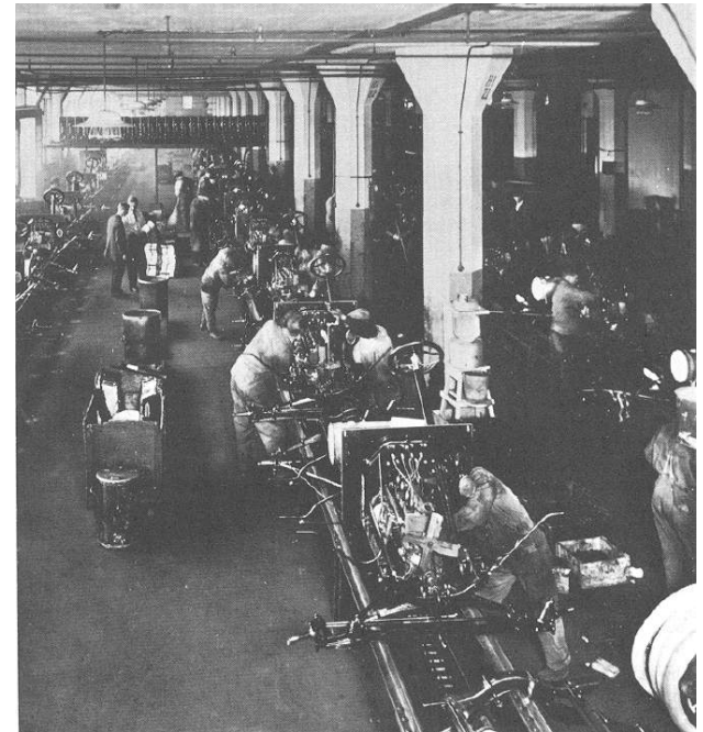
Ford's Moving Assembly Line
