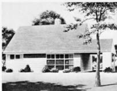
REAR VIEW OF ALL HOUSES
