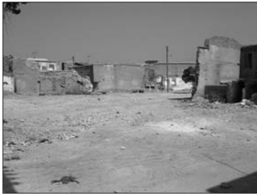
Fig. 4 A demolished house in one of the old neighborhoods.
