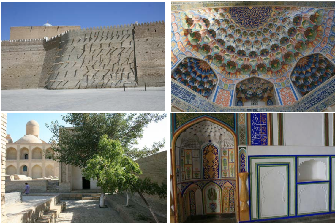
Figure 5: Examples of recent restoration of historical monuments in Bukhara. Top left: Restoration of the Ark Citadel - the oldest historical monument in Bukhara. In April 2011, part of the Ark’s wall collapsed. The collapse was due to the poor previous restoration of the same area in 2010. In both cases, there had been a serious violation of building techniques and materials while restoration. According to its original construction, the Ark was structurally supported by logs running through the thickness of
