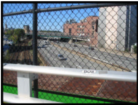
Figure 22. Massachusetts Turnpike and Commuter Rail; view from Brookline Ave. Air rights could be a major influence on the square.
