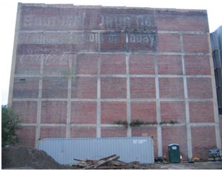
(The regular concrete frame structure on the Lerner Building offers opportunities to remove the brick infill for more light and to maintain a flexible and open floor plan within the structure. Image courtesy of Urban Focus team)
