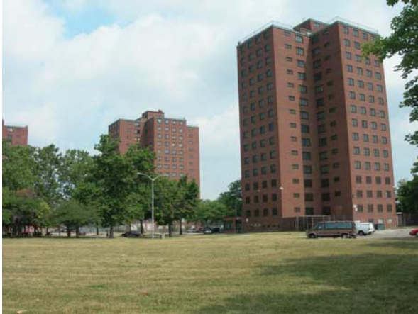
Figure 6. Many older blocks were cleared and consolidated for urban renewal programmes such as this public housing directly north of downtown Detroit.
