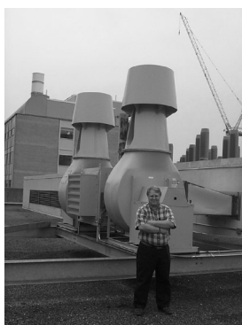
ChE Facilities Manager Steve Wetzel with new roof mounted dual-exhaust blowers.
