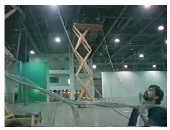
Figure 6: Screen grab of the construction of the Interop trade show's INTEROPnet (or ShowNet). The routing and bridging equipment used to construct the show network was estimated to have been as much as a major corporation would use to supply offices in fifteen or twenty cities.<sup>34</sup>
