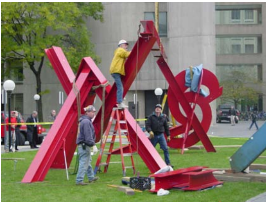
Artist Mark di Suvero (on ladder) and a team of assistants spent the better part of a day installing this sculpture on the lawn near the Stata Center.
