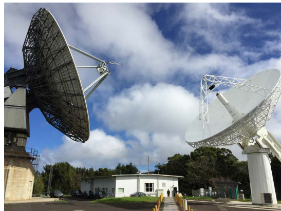
The first fully operational VGOS system installed at Koke'e Park on the island of Kauai. The new VGOS antenna is on the right.
