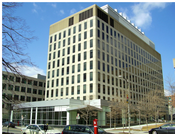
Fig. 6: ISN headquarters and labs occupy the fourth and fifth floors of 500 Technology Square (NE47) in Cambridge, MA.
