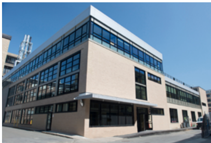
Building 31, home of the Gas Turbine Laboratory and autonomous systems research, has undergone a $52 million renovation.
