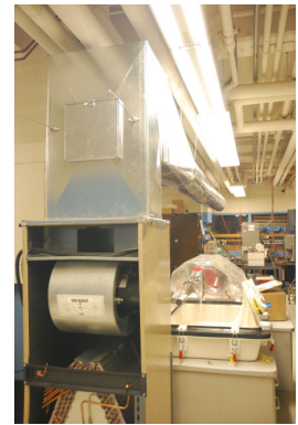
Fig. 13. Additional view of ducting apparatus.
