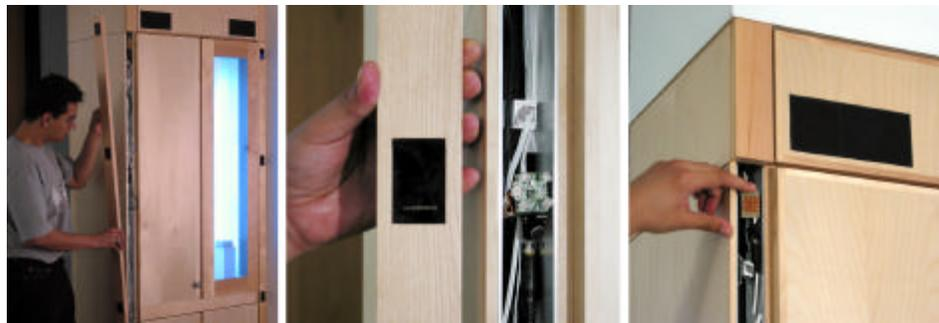
Interior Infill Cabinetry Component with Integrated Technologies
