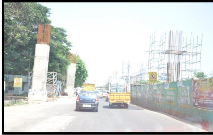
Fig.1 View of Work Zone Section with Reduced Width along GST Road
