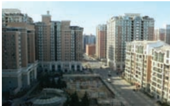
Fuguiyuan > Photograph of towers and flats Source Jie Bai.
