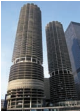
Marina City Towers, Chicago > 19 floors of exposed spiral parking ramp, housing nearly 900 parking spaces form the base of each of these 179-meter tall buildings. Source: supernova9@flickr.com.
