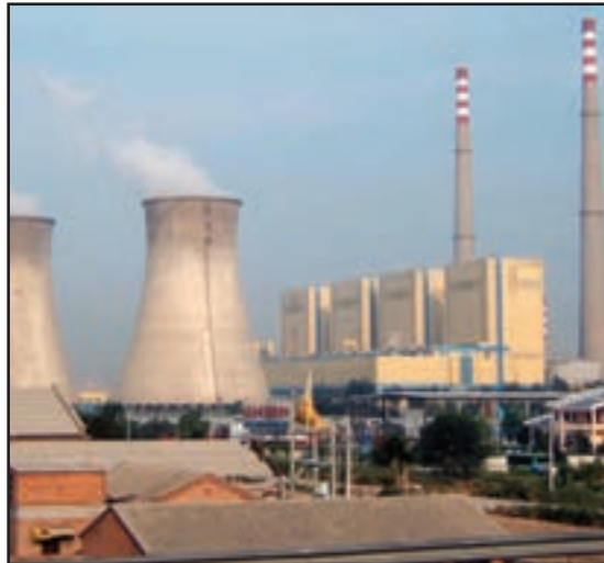
Energy Provider > District heating/cooling networks are fueled by waste heat from power plants, which are often sited near urban development in China. Source: Brett Arnett at flickr.com.
