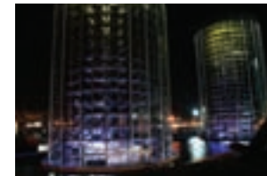
Volkswagen Autostadt, Germany > New cars are delivered to their owners via a 60-meter tall auto elevator at this Volkswagen factory in Germany. The elevator transports the cars at a speed of 1.5m per second. Source: New York Times.
