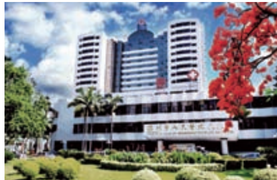
Shenzhen People's Hospital > The biggest healthcare facility with 1,000 beds on 9ha of land. Source: Shenzhen People's Hospital
