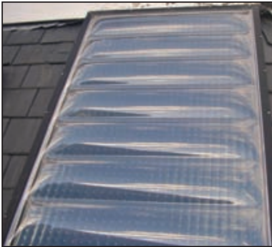
Solar Power > Solar hot water panels can be installed on building rooftops to heat water that can be used by residents. Excess hot water can be “sold” to the district heating/cooling network. Source: nenorufus.at/flickr.com
