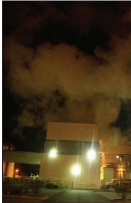
MIT Cogen Plant > Steam escaping from the MIT Cogen Plant, which serves all of MIT through a network of piping integrated into tunnels or building infrastructure. Source: Frank Hebbert.
