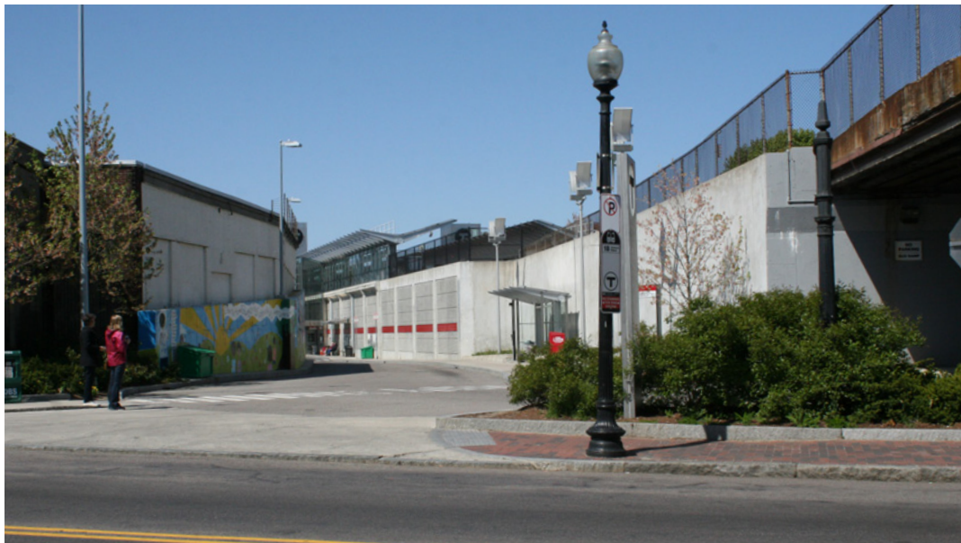
Figure 5.12. Renovated busway and pedestrian improvements at Fields Corner Station
