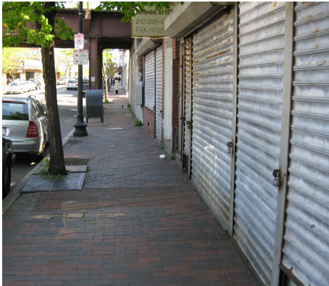
Figure 5.20. Existing conditions of eastern façades on Dorchester Avenue.
