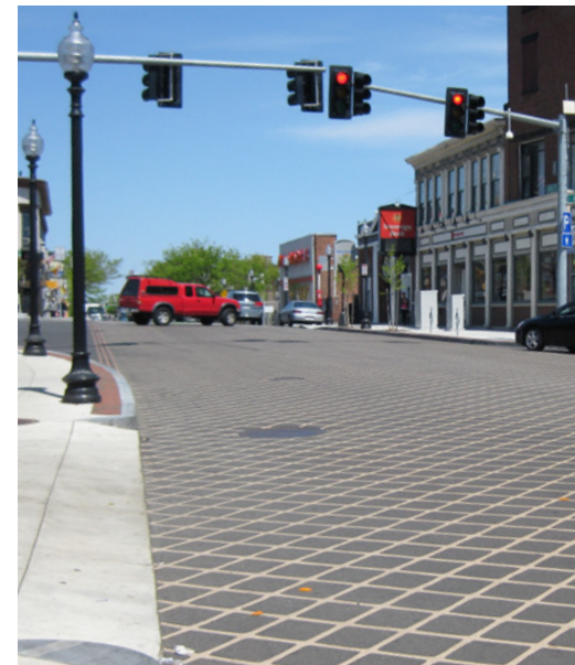
Figure 5.13. Duratherm-treated intersection at Dorchester and Adams
