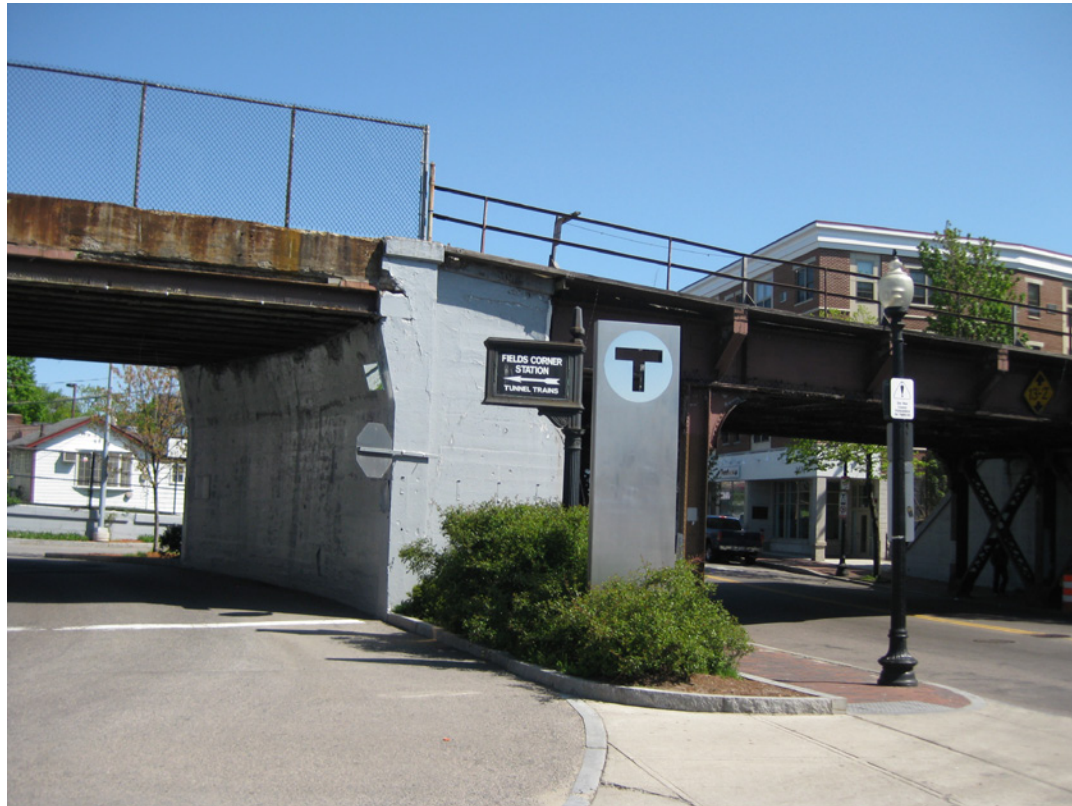
Figure 5.17. Signs indicate the presence of Fields Corner station, but the barrier of the hedge and the lack of a clear pedestrian path (the crosswalk is behind the camera) downplay the connection.
