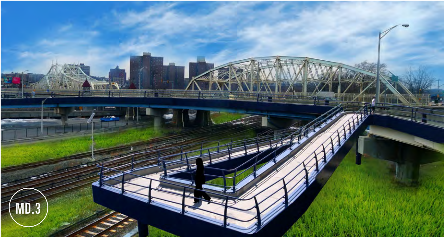
The dangerous Macombs Dam Bridge crossing is improved by adding a pedestrian and bicycle underpass below the bridge.
