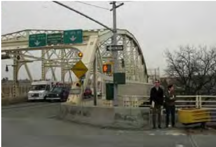
Pedestrians have to cross three times to travel north or south along Sedgwick Avenue at the intersection with the Macomb's Dam Bridge.
