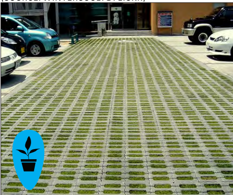
PERVIOUS PAVERS PREVENT WATER RUN-OFF AND MAKE AN INTERESTING ALTERNATIVE TO ASPHALT.
