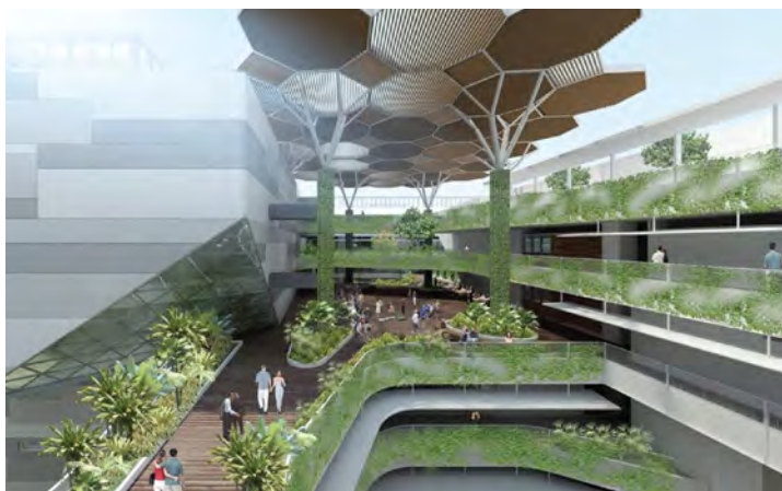
▲ Buildings at Nanyang Technological University (NTU) received BCA Green Mark Platinum Awards in 2016. Image: NTU
