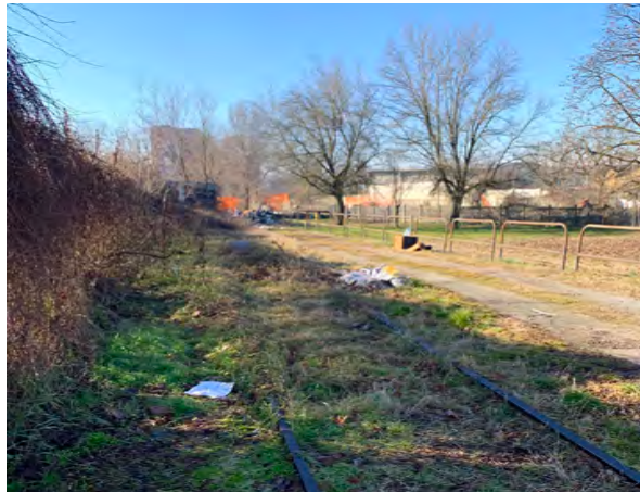
▲ Unmaintained edges along the rail
