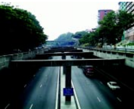
View of Central Expressway.
