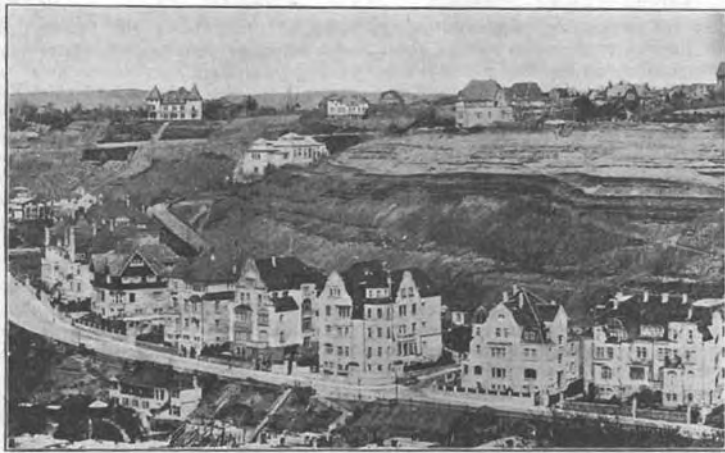
A NEW "ONE SIDED" STREET ON A STEEP HILLSIDE. DISTRICT BUILDING REGULATIONS PERMIT NO BUILDINGS ON DOWN HILL SIDE TO OBSTRUCT THE VIEW.
