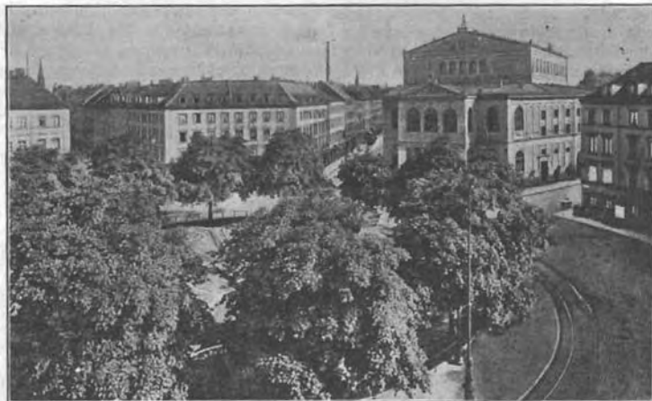
TYPE OF DISCARDED ROND POINT TREATMENT INTERRUPTING TRAFFIC ROUTES AND ENCOURAGING CONGESTION BY NEEDLESS CONCENTRATION OF THOROUGHFARES.
