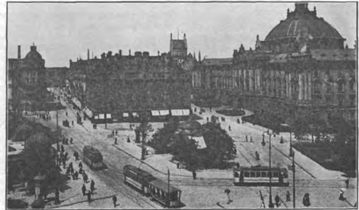
VIEW ACROSS A RING-BOULEVARD AT THE POINT WHERE IT IS INTERSECTED BY TWO RADIAL THOROUGHFARES.
