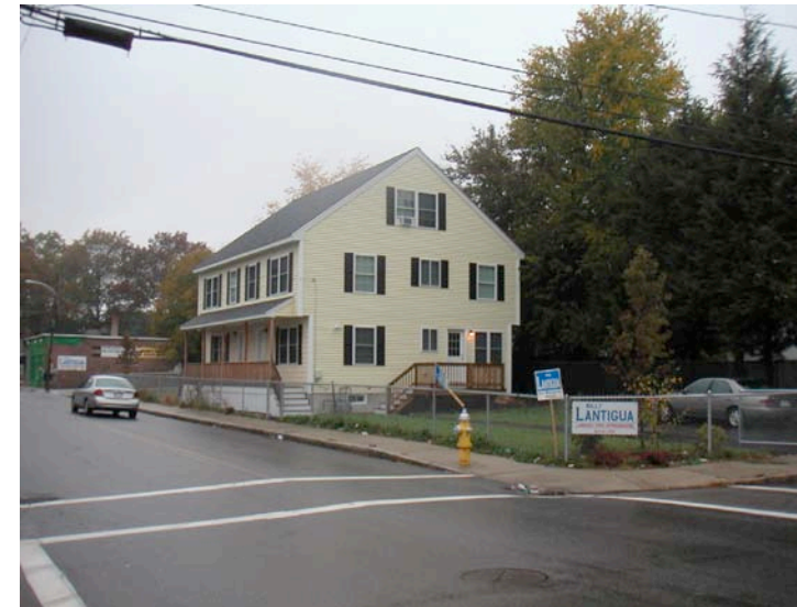
125-127 Park Street: Disposed to Bread and Roses Housing, Inc., November 2004
