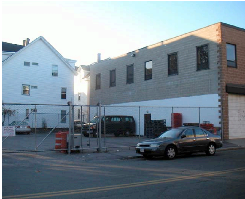
410 Hampshire Street: Disposed to Lazarus House, March 2001
