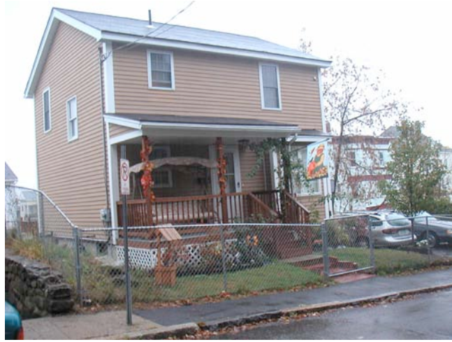
19 Bevel Street: Disposed to Habitat for Humanity, October 2002
