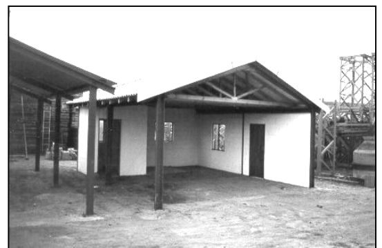
Photo 2-1: South African version of a roof house, Durban
