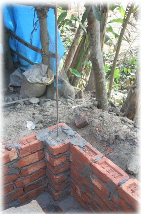
Design features such as concrete reinforced brick columns considerably add to the strength of the houses.
