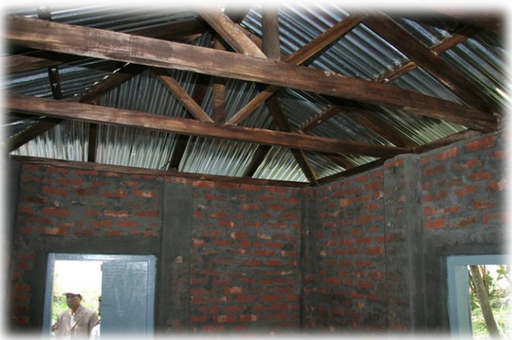
Strong wooden roof trusses offer resistance to high winds
