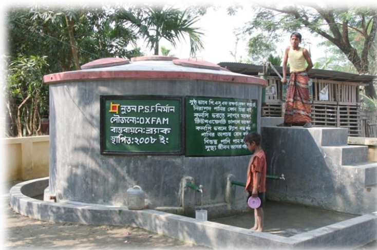
BRAC has constructed 252 pond sand filters throughout the Sidr affected region with OA/ON support, providing safe water to more than 250,000
