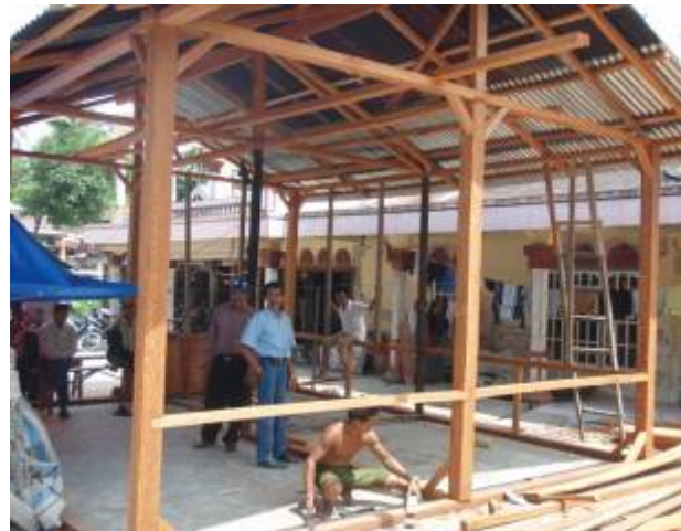
Community start constructing
