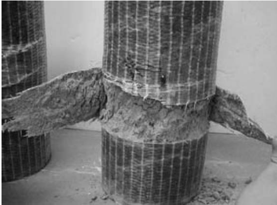
Fig. 1. Local concrete crumbling [2].
