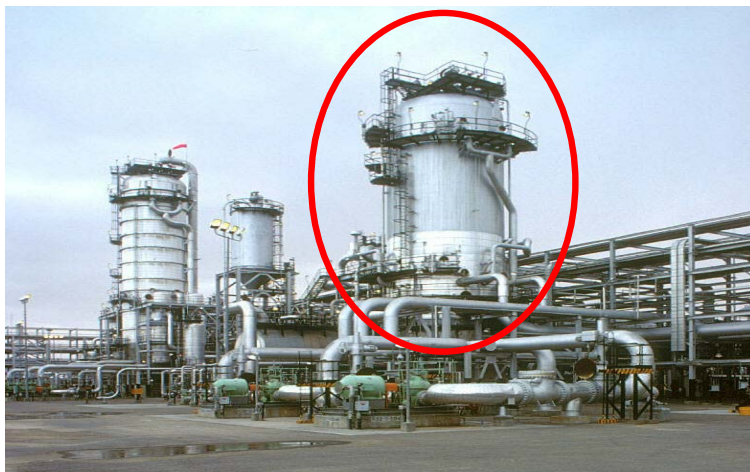
Figure 10: Fluor's DGA Plant in Uthamaniyah, Saudi Arabia has absorber (center-right) with a large diameter
