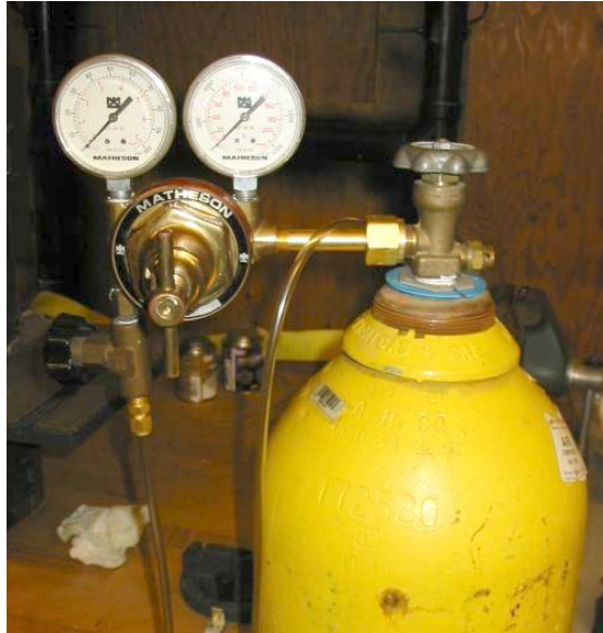
Figure 3-5: Compressed air supply tank and regulator.
