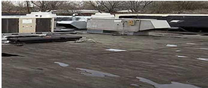
modified bitumen roof
