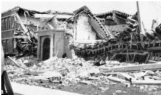
Figure 2. Jefferson Junior High School following the Long Beach, CA earthquake of 1933. Courtesy of the Portland Cement Association.
