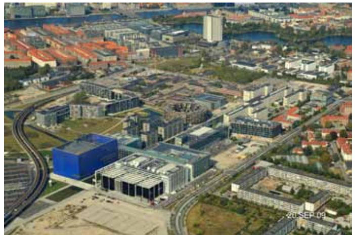
Ørestad Nord seen from the east overlooking the City and Harbour of Copenhagen. (courtesy Ørestad Nord Gruppen)
