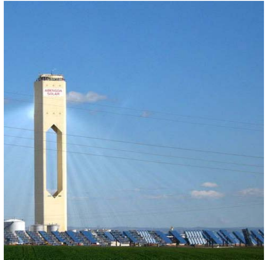
PS-10, 11MWe peak, Image courtesy of N. Hanumara
