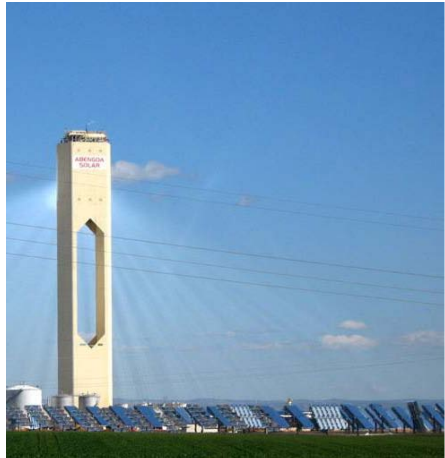
PS-10, 11MWe peak, image courtesy of N. Hanumara
