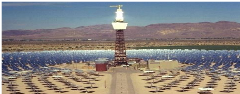
Conventional CSP “Power Tower”
