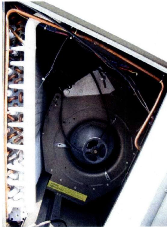
Figure 2-2: Picture of broken mount for fan motor in a field-installed AHU, from [31].
