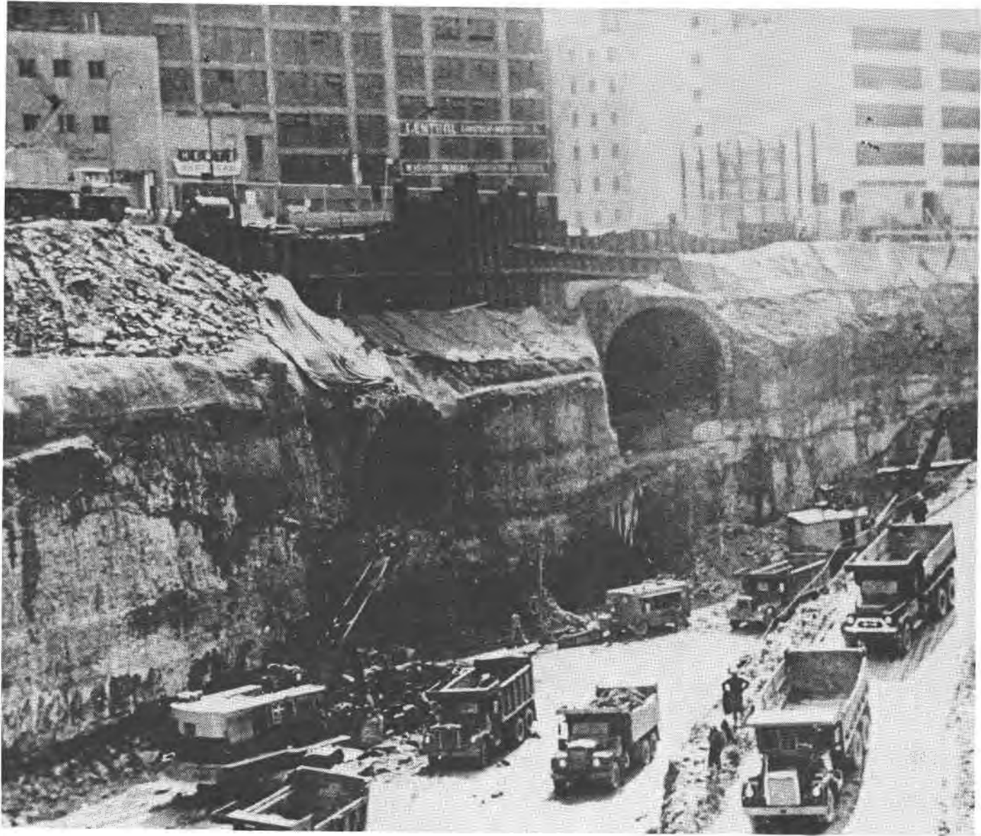
FIG. 3. Grant's Hill Tunnel, lower left, and Pennsylvania Railroad Tunnel, upper right, encountered while excavating for foundation of the U.S. Steel Building (courtesy of the Historical Society of Western Pennsylvania).
