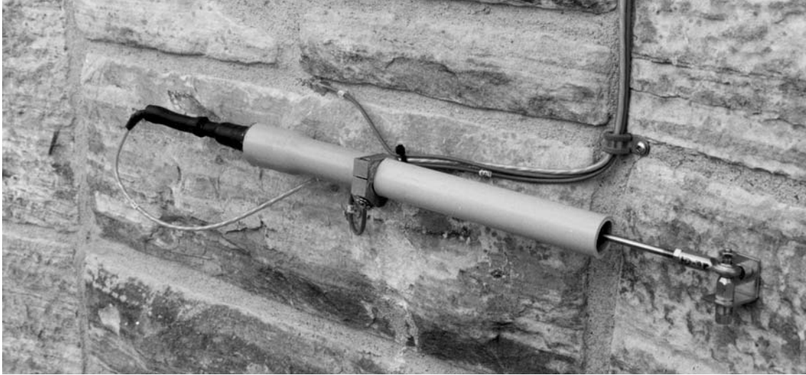
Figure 2. Linear variable differential transformer (LVDT) displacement sensor on the northwest face of the northwest buttress of the Peace Tower. A grey PVC tube covers the stainless steel LVDT to reduce its visibility to the public. A thermocouple temperature sensor glued to a mortar joint right above the LVDT measures surface temperature of the masonry.
