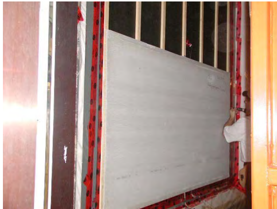
Figure 14 - Installation of cement board (Location 7)
