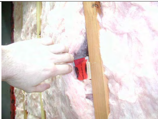
Figure 20 - Installation of ACR sensor in stud cavity
