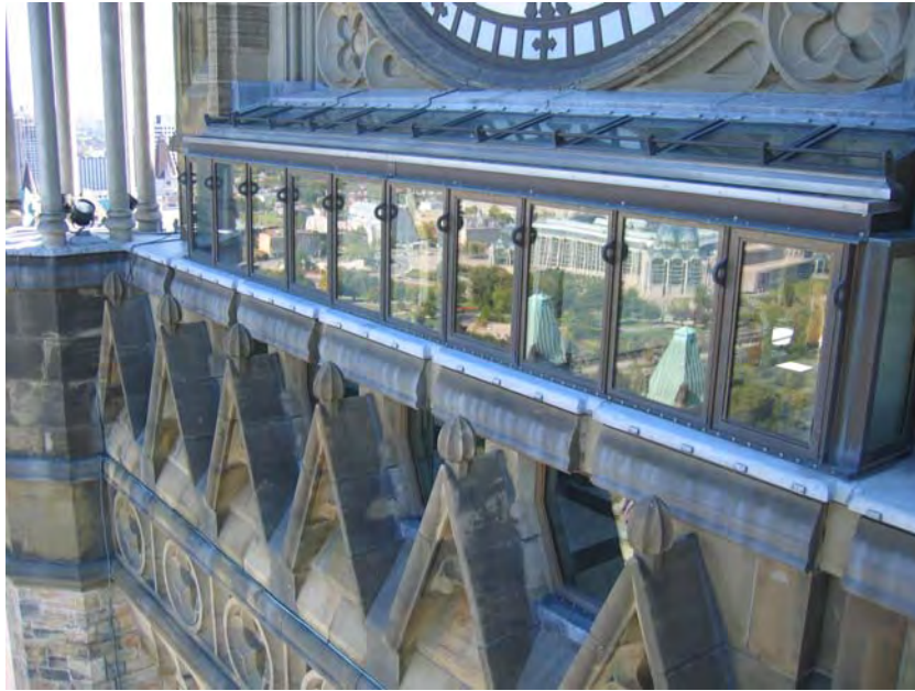
Figure 9. Photo showing dampness of the north façade at the Observation level. Notice the good condition of the Wallace stone and the mortar joints. The gray stain is a result of run-off water from the lead flashing above.
