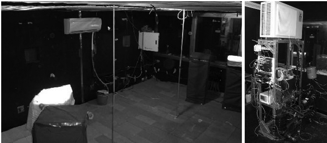
Figure 3. Left: Test office chamber with concrete radiant floor, simulated internal loads, and a conventional split-system air conditioner indoor unit. Right: Low-lift chiller in the climate chamber.
