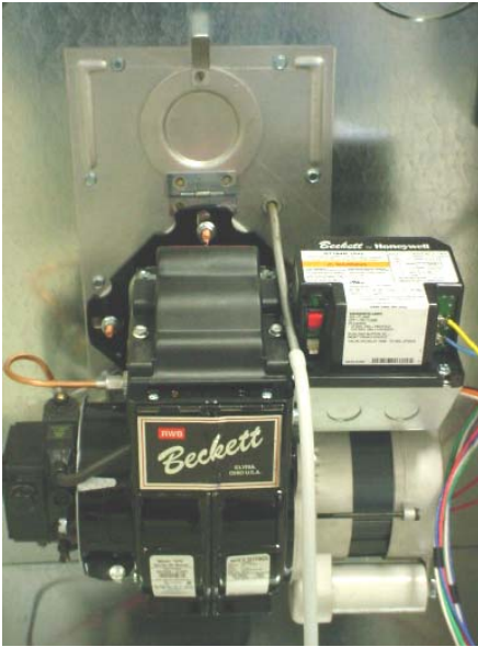
Fig. 5: Checking Over-Fire Draft.
