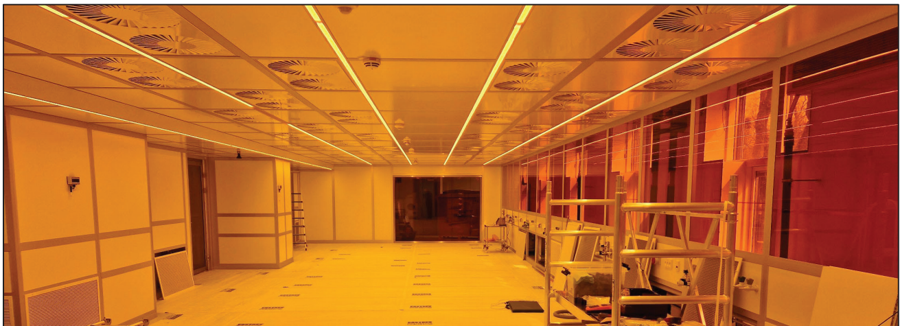
Figure 1: The PolyFabLab ISO 7 cleanroom during the last stages of installation.
